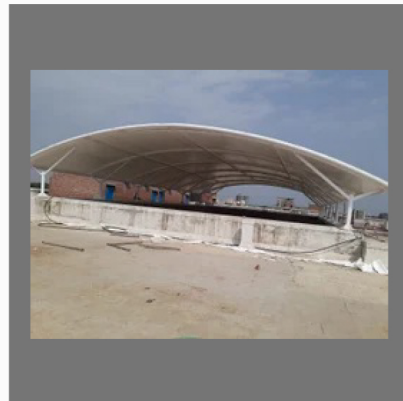
Tensile Roofing Structure
