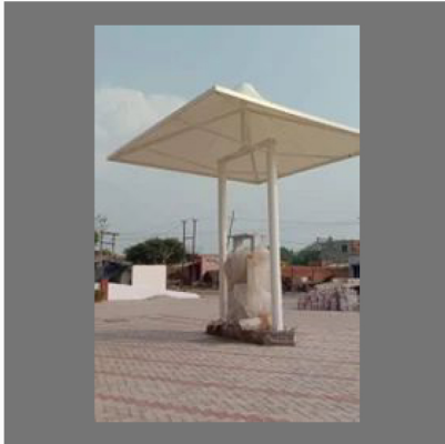
Car Parking Tensile Structure
