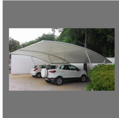
Car Parking Tensile Structure
